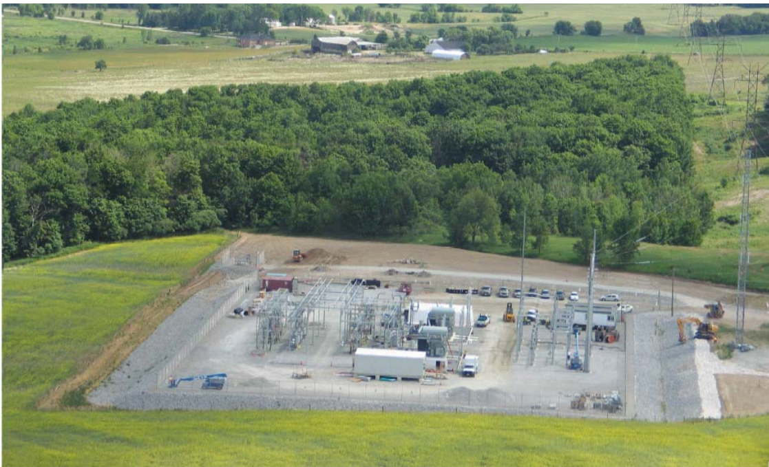
Figure 1-4 Construction of a TS similar to the proposed Leamington TS
