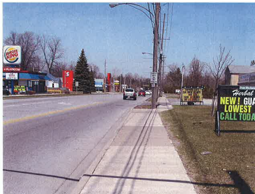
Typical View of existing conditions on Malden Road, within Northern, “Urban” Area, or “Town Centre” (looking north). Note inconsistent alignment of sidewalk.
