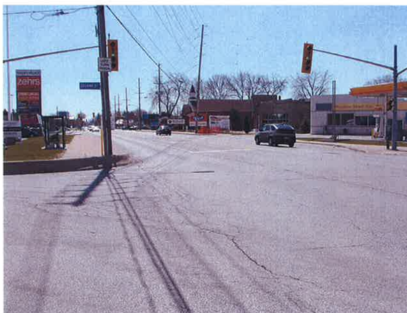
View of existing conditions on Malden Road, within Northern, “Urban” Area, or “Town Centre” (looking south at Delmar Street.) Note unmarked crossings and pedestrian barrier and varying surface-types on sidewalk.
